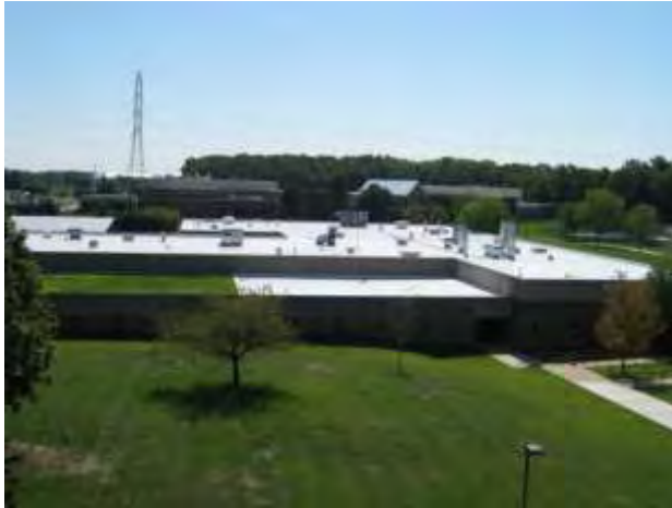
Figure 29: Roof view with vegetated area
