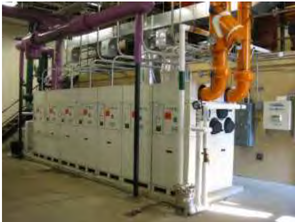
Figure 31: Modular geothermal water-to-water heat pump
