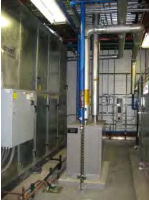
Figure 38: Humidification equipment
