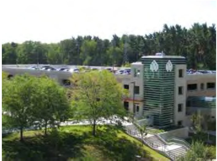
Figure 9: Campus Green Parking Structure
