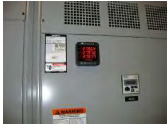
Figure 7: Electrical sub-meter
