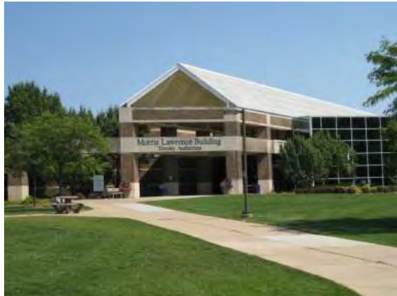
Figure 27: Morris Lawrence Building
